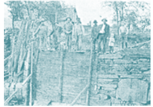
Workers rebuilding one the dams on Powell Brook that powered the two mills (probably between 1910 and 1917).
